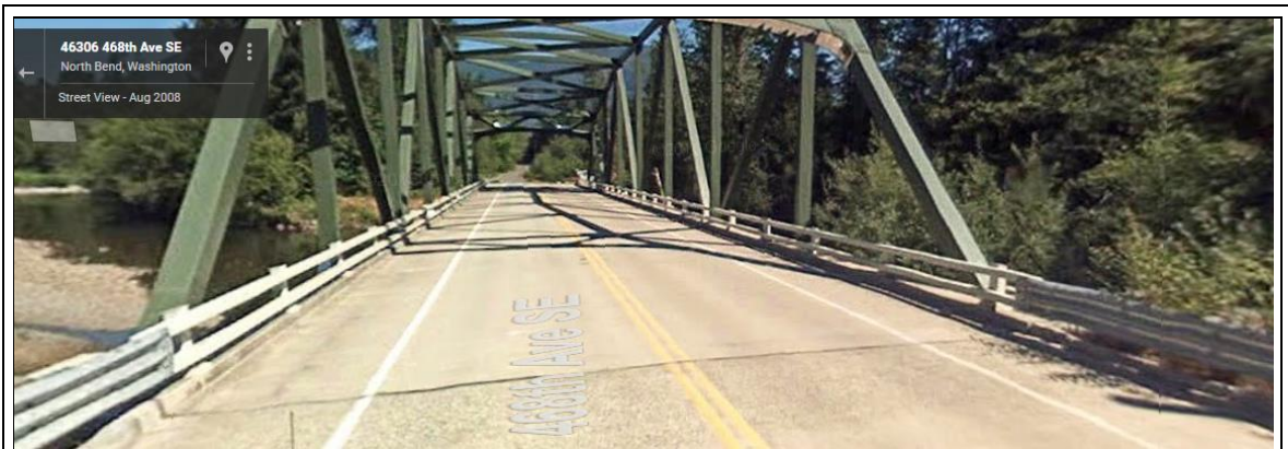
Pre-installation view 08/ 2008 (Google Maps satellite image)
