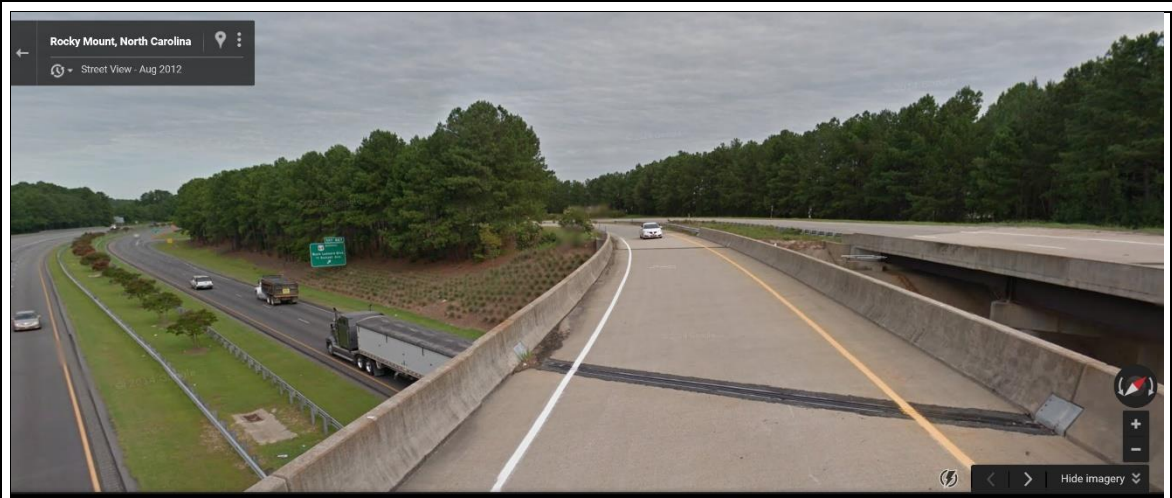
Google Image Pre-Installation 2012
