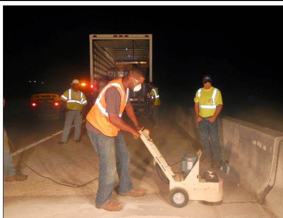
Bump grind for rideability 15 minutes after set
