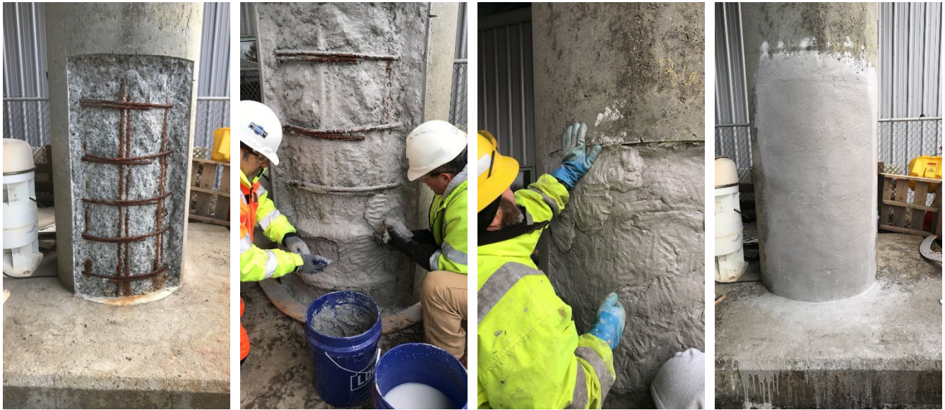
Extensive bridge column repairs were performed by the contractor on this long-span bridge using F1-VO in 2020
