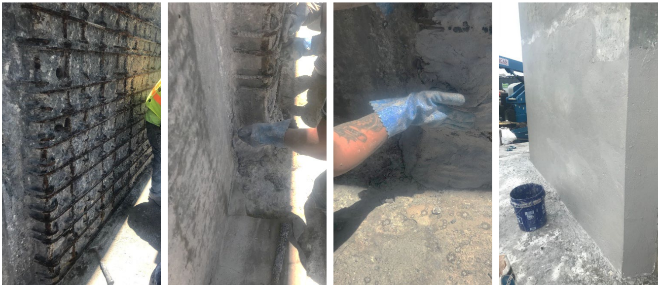
Structural wall repairs were performed by the contractor using F1-VO [MALP] in 2020
