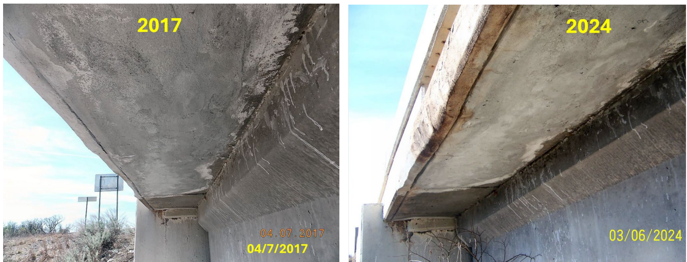
Inspection by Oklahoma DOT after 7 years shows no corrosion and no delamination of the Phoscrete repair.
