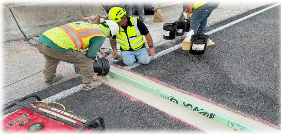
Figure 10 Phoscrete Formula 3-HC is an approved bridge expansion joint nosing material. Installation was performed by a contractor for FDOT on I-75 - Alligator Alley (2024).
