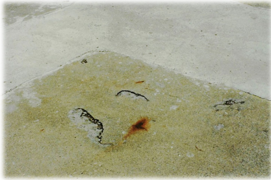
Figure 5 Halo/Ring Anode Effect: Corrosion forms adjacent to the patched concrete.
