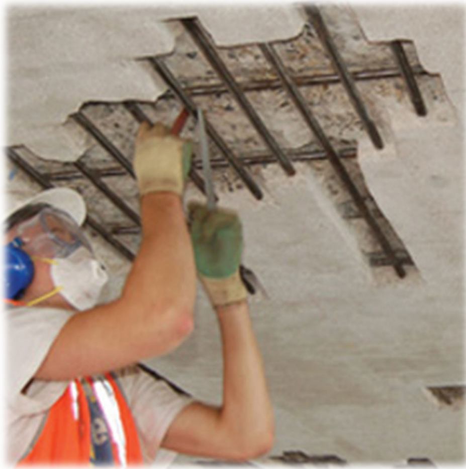
Figure 7 Site preparation for nitrites and zinc anodes requires extensive demolition under the rebar plus rust removal.
