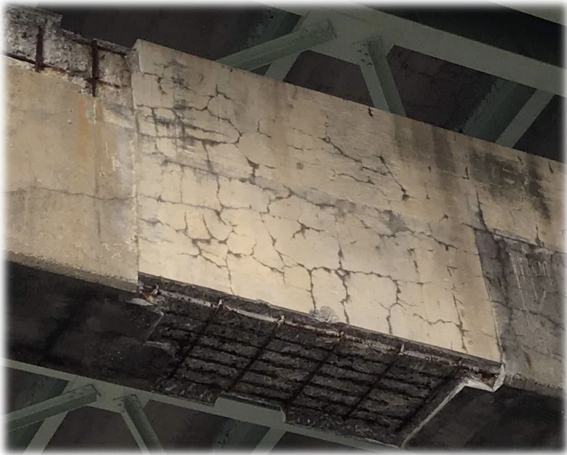
Figure 3 Crack propagation due to rust expansion on a bridge beam in Rhode Island, 2020
