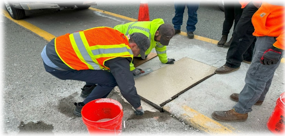
Figure 9 Phoscrete Formula 1-HC winter pavement repair at MassPORT (2024).
