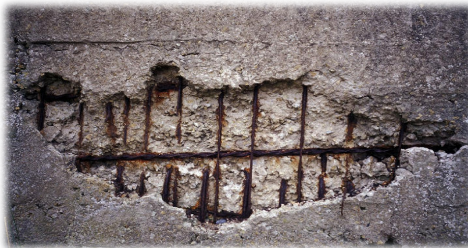
Figure 2 Chloride-induced corrosion and spalling in concrete.
