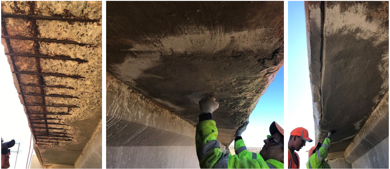
Phoscrete F1-VO [MALP] was installed by hand-packing, trowel finishing in 2017 with minimal site preparation.
