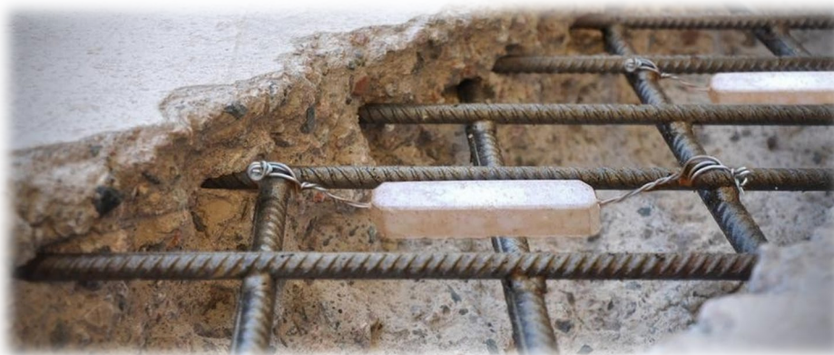
Figure 6 Galvanic cathodic protection with zinc sacrificial anodes.
