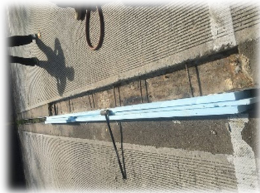
Use Foam Board to Establish Expansion Joints
