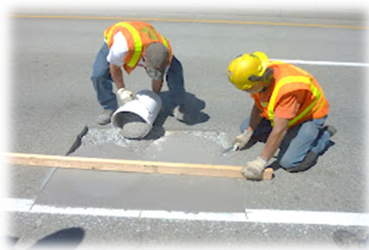
Bridge Deck Spall Repair
