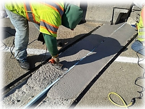
Expansion Joint Header Installation
