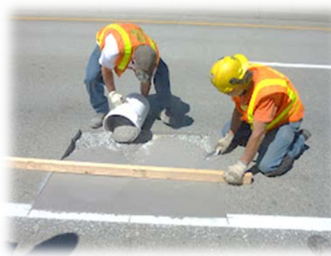
Bridge Deck Spall Repair
