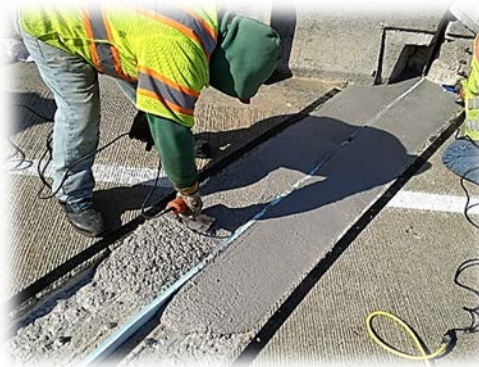
Expansion Joint Header Install
