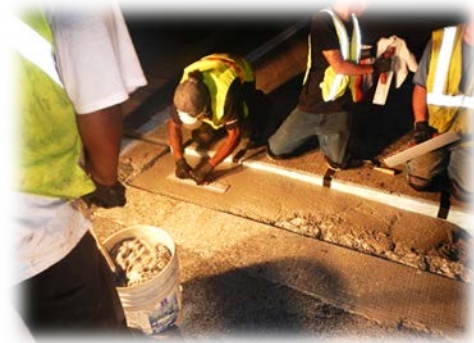
Use Blue Board to Establish Expansion Joints
