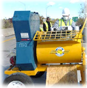
Paddle-Style Mortar Mixer with plywood to direct material
