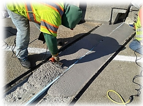
Expansion Joint Header Installation
