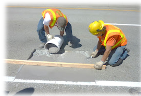
Bridge Deck Spill Repair
