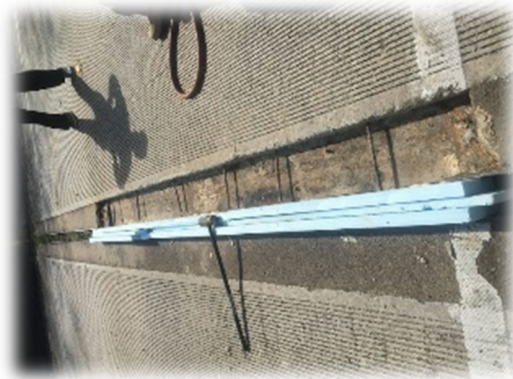
Use Foam Board to Establish Expansion Joints
