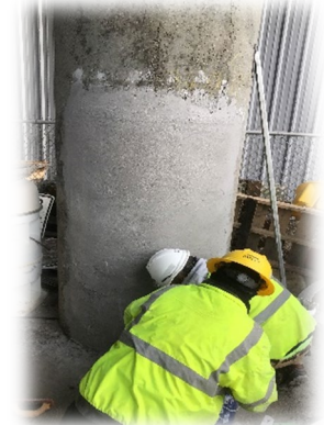
Vertical Column Repair
