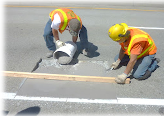
Bridge Deck Spall Repair
