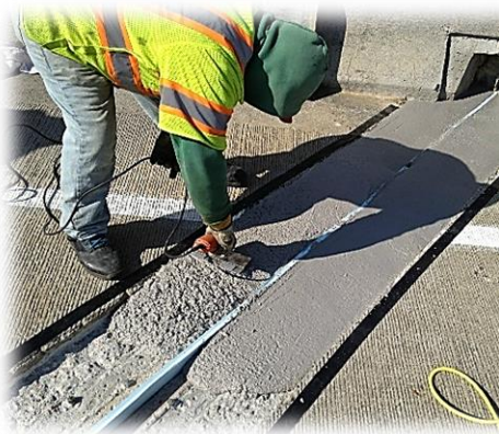
Expansion Joint Header Installation
