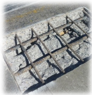
Deck Spall Ideal Site Preparation
