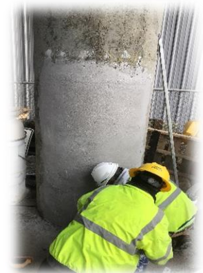
Vertical Column Repair
