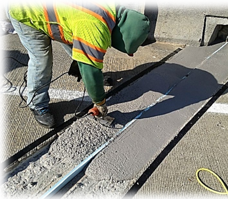
Expansion Joint Header Installation
