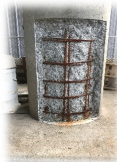
Vertical Column Site Preparation
