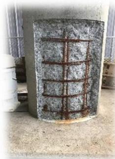
Vertical Column Site Preparation
