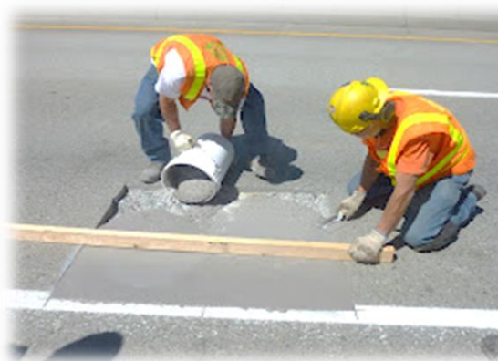
Bridge Deck Spall Repair
