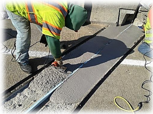
Expansion Joint Header Installation
