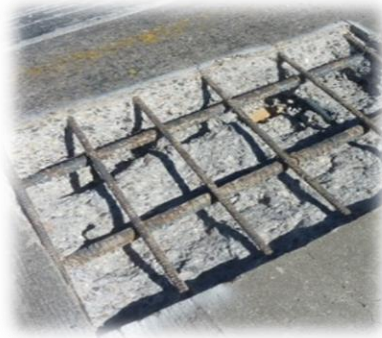
Deck Spall Ideal Site Preparation
