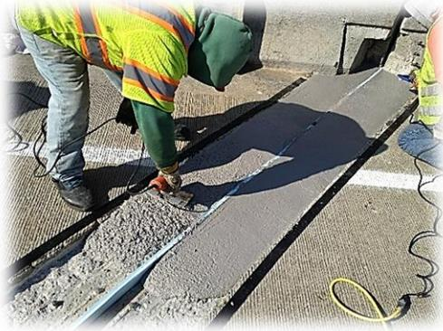
*Expansion Joint Header Installation*
