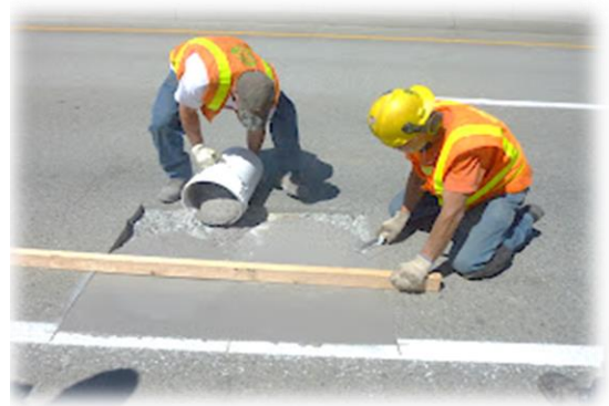
Bridge Deck Spall Repair
