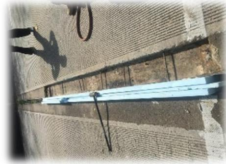
Use Foam Board to Establish Expansion Joints
