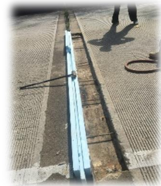
Use Foam Board to Establish Control and Expansion Joints
