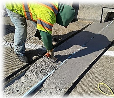
Expansion Joint Header Installation
