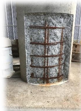
Vertical Column Site Preparation
