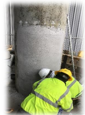
Vertical Column Repair
