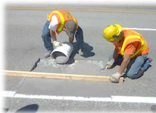
Bridge Deck Spall Repair
